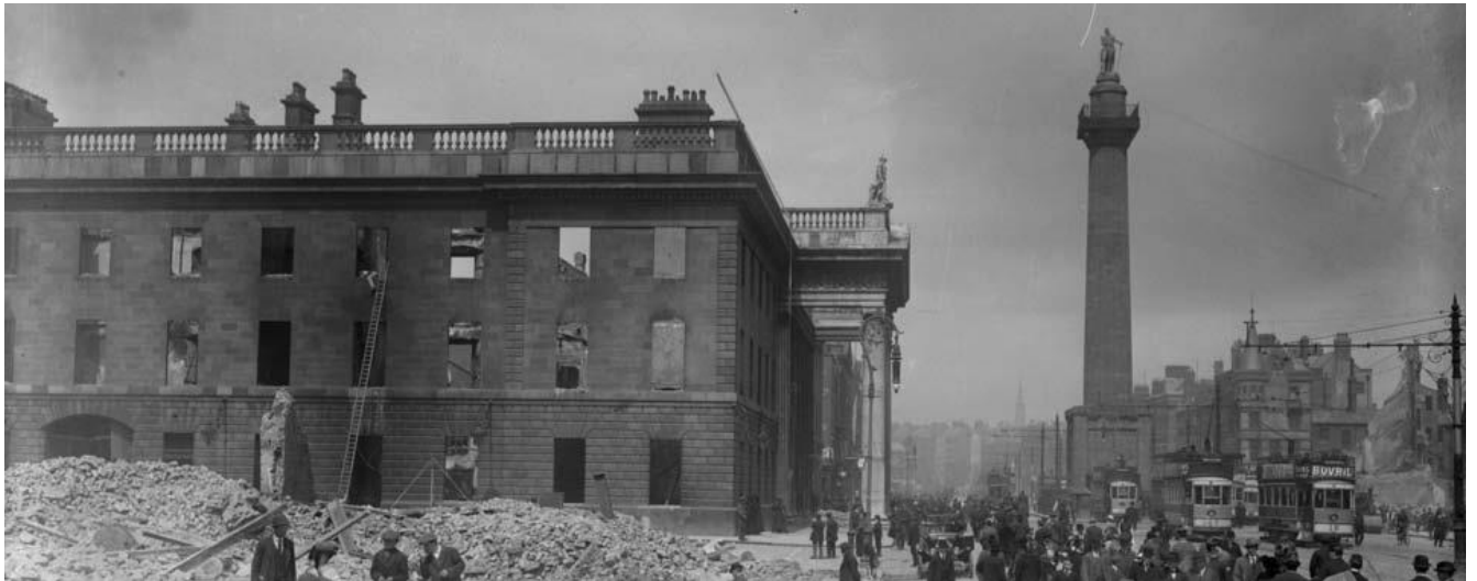
The Dublin GPO building after the rebellion
